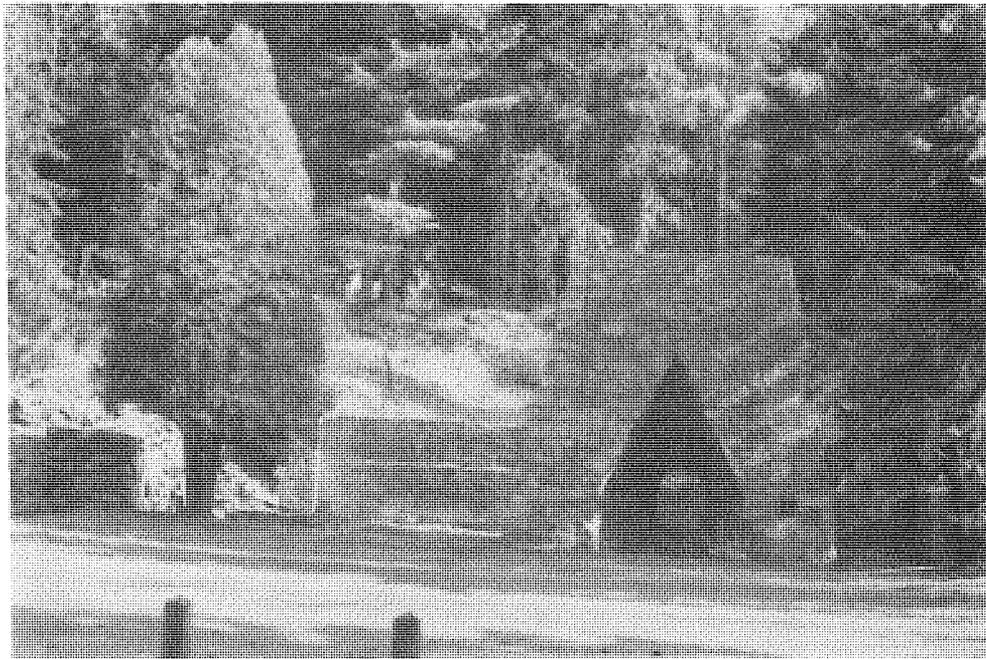
Figure 22. Greenwood Furnace Stack No. 2 at Greenwood Furnace State Park. Constructed in 1866 and restored in 1935, this was a hot-blast charcoal furnace in which the escaping exhaust gases were used to heat the air blast. The ruins to the left are the remains of Stack No. 1, a cold-blast charcoal furnace erected in 1854 (?). These furnaces used a mixture of Clinton "fossil" ore from nearby Brush Ridge and "brown hematite" ore from Kishacoquillas Valley on the other side of Stone Mountain.
