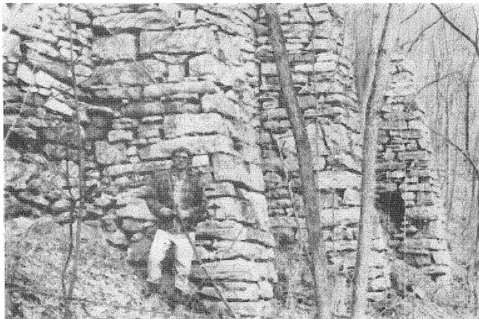
Figure 20. Dolomite-block buttresses of the charcoal house at Mount Etna iron furnace plantation. The ruins of this structure are located about 60 m east of the old blast furnace. William I. Richardson provides scale.
