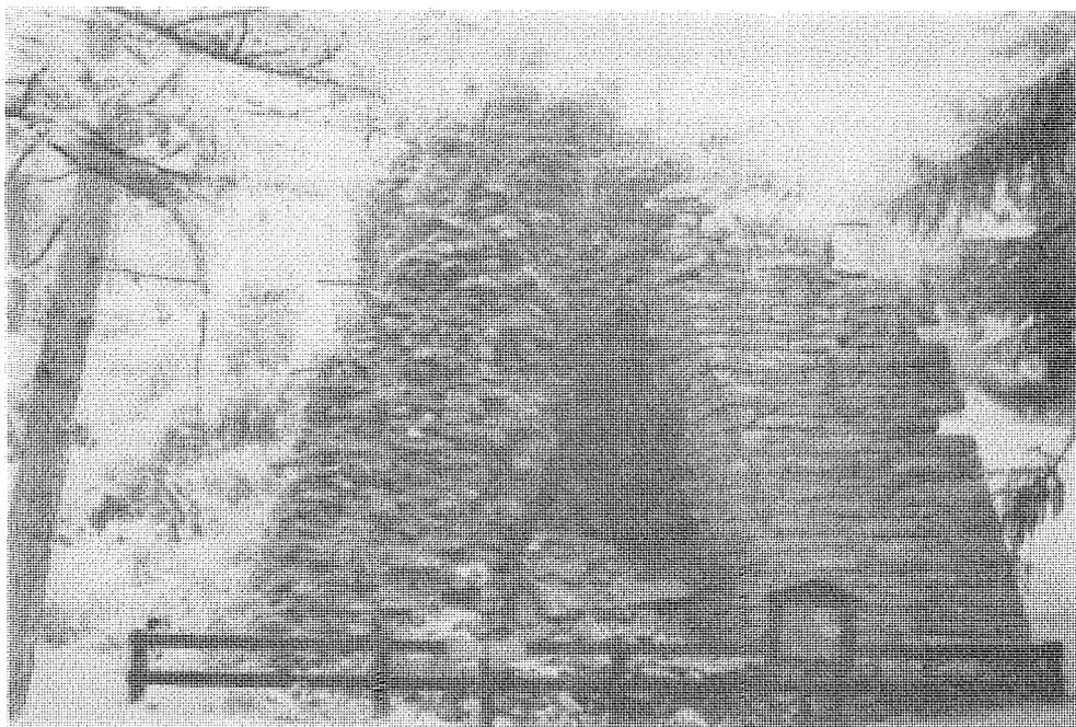
Figure 23. Sandstone stack of Paradise furnace behind park office at Trough Creek State Park, Todd Township. Erected by Lubin Trexler in 1832, this furnace used "Mauch Chunk" limonite ore during its two periods of operation 1832 to 1845 and 1860 to 1868. The ironmaster's mansion on the hill overlooking the furnace is currently used as the Park Superintendent's residence.
