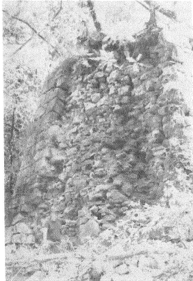
Figure 21. Ruins of Elizabeth furnace near Pinecroft. Like many of these old furnace stacks, this one has collapsed over the broad work arch (where the molten iron was drawn from the furnace). Note the unmortared limestone block facing on the exterior, and the random, unsorted material forming the middle layer of the furnace. The inner brick lining is not exposed. The author provides scale.
