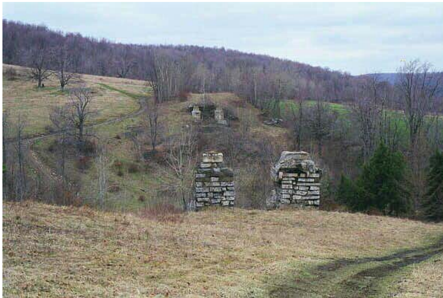
Figure 30. View north across the valley of Bucks Creek, showing the stone pier-foundations of the Erie/D&H railroad-trestle (wood, 1870; steel, 1888) that once crossed the valley just upstream of the falls.
