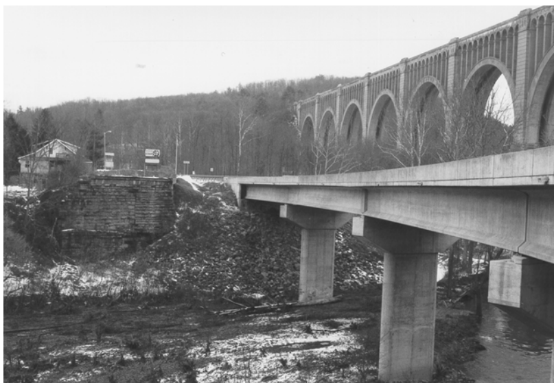
Figure 95. The “Bridges of Tunkhannock Creek.” View north from STOP 6, showing (left to right) the abutment of the old DL&W Railroad bridge (1850’s, also used after 1915 for the original highway bridge), the new US 11 bridge (1990), and the Tunkhannock Viaduct (1915).
