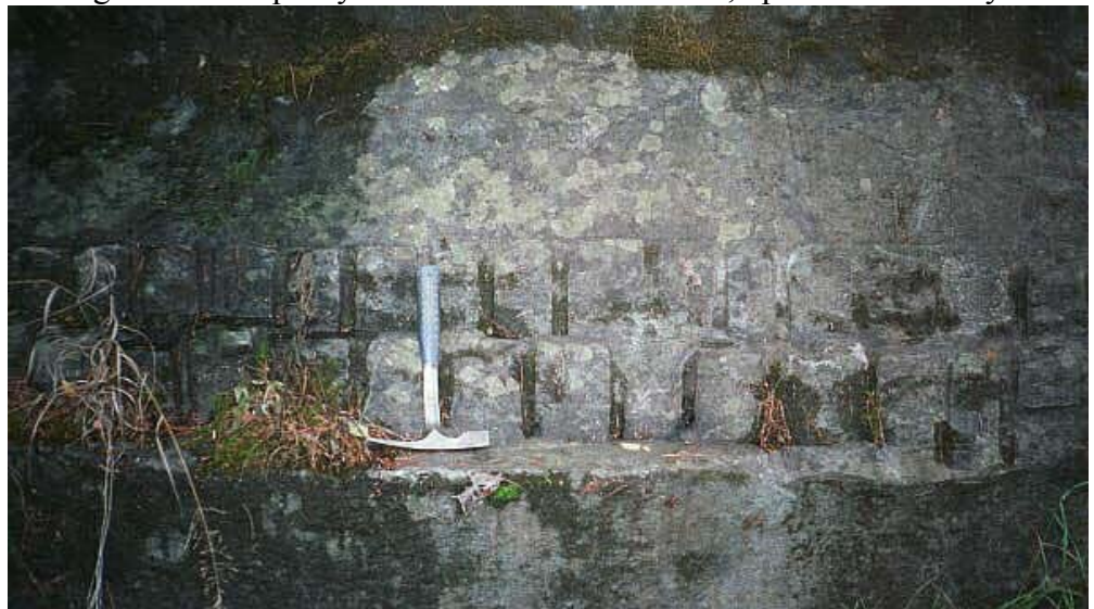
Figure 62. Star-drill marks in massive, basal sandstone at STOP 2, Site A. Hammer is 11 inches long.
