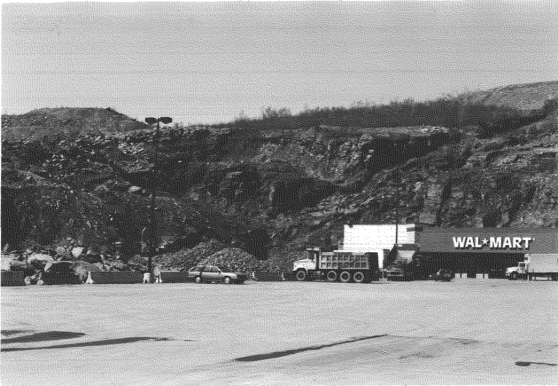
A. Distant view of the WAL-MART rockslide (STOP 9). Even from across the parking lot the intensely disturbed nature of the rock strata is evident.
