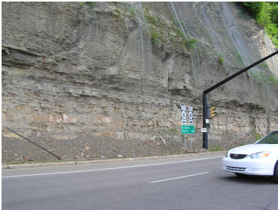
Figure 4. Recent photograph of the PA Route 8 roadcut at Oil City.
