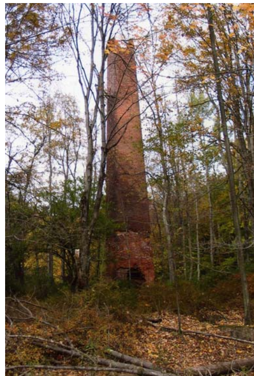
Figure 45. Tall brick chimney marking the site of the Jamison City tannery.
