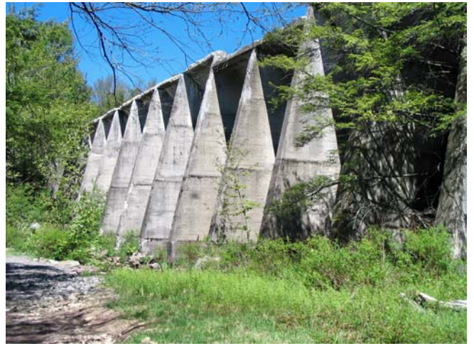
Figure 1-40. Downstream face of Lake Leigh Dam, showing concrete-curtain construction.
