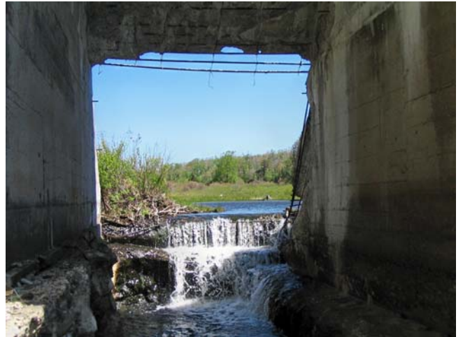
Figure 1-42. View of Lake Leigh wetland through one of the demolition holes.
