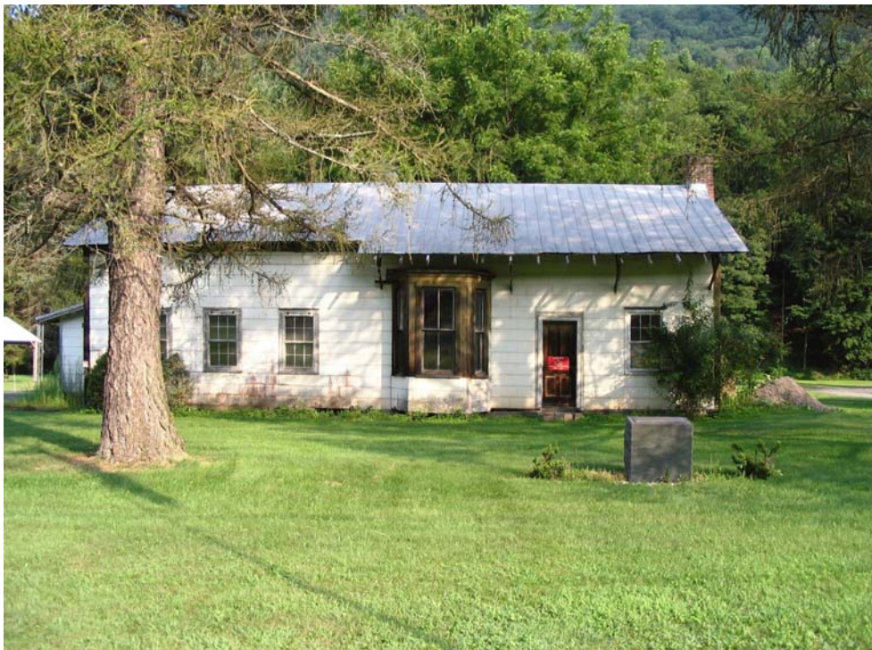
Figure 33. The former Bloomsburg and Sullivan Railroad station (1889-1926) in Jamison City.
