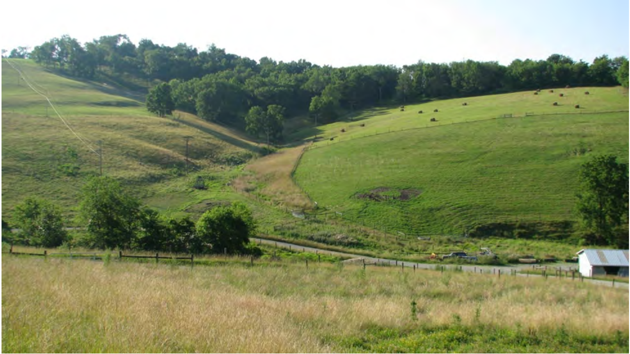
Figure 12. Landslide areas on the left lower slope, the right lower slope.
